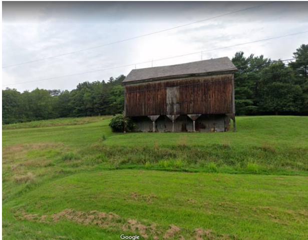
FIGURE 18: THE HISTORIC BARN LOCATED ON THE PROPERTY ACROSS FROM LINBROOK PARK. IMAGE: GOOGLE EARTH.
